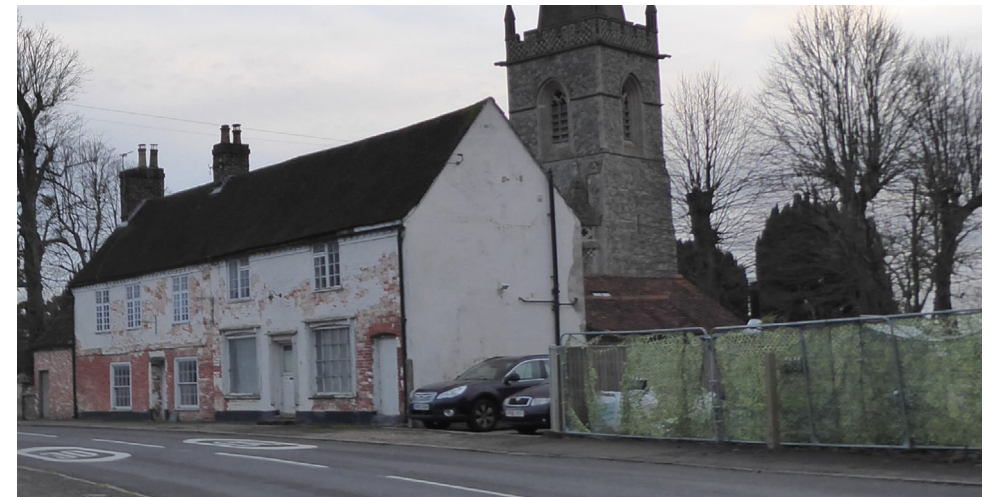
Figure 43 Church Cottage in state of disrepair and Heras fences at the boundary of Crown House
