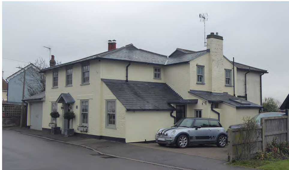
Figure 28 The Saltings, Manor Road
