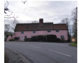
Figure 15 Grade II Listed Crown House
