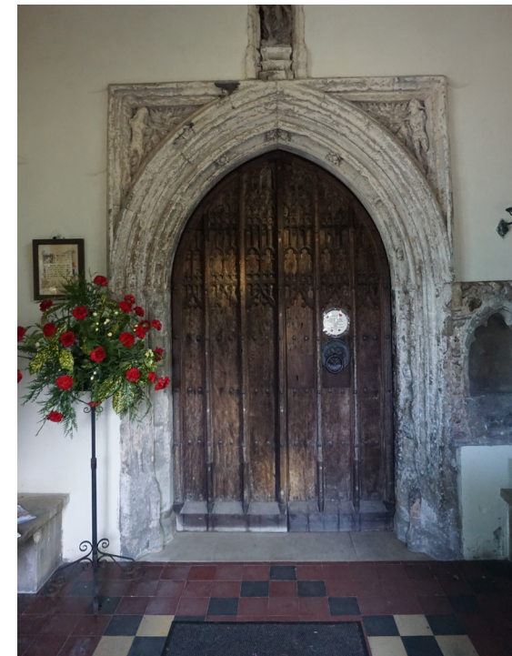
Figure 8 St Mary's Church door
