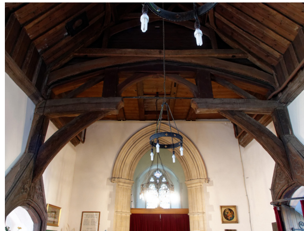
Figure 22 Fourteenth century hammerbeam truss at St Edmund's Church Pevsner remarked: "The tracery detail of the gables is clearly of the fourteenth century, and not too late in the century either, and thus this truss is earlier than the hammerbeam roof of Westminster Hall, in the text books still called 'the earliest in existence'
