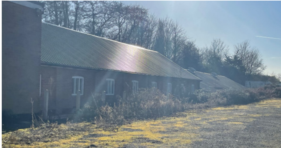
Figure 31 Ardleigh Studios (former goods sheds)
