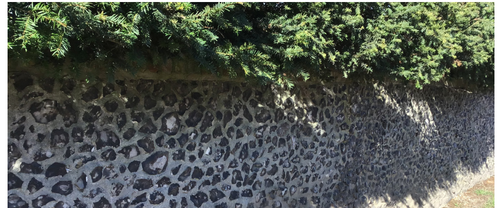
Figure 27 Flint rubble boundary to The Old Rectory
