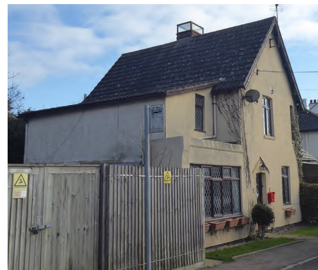
Figure 58 Ivy Cottage on Rectory Road
