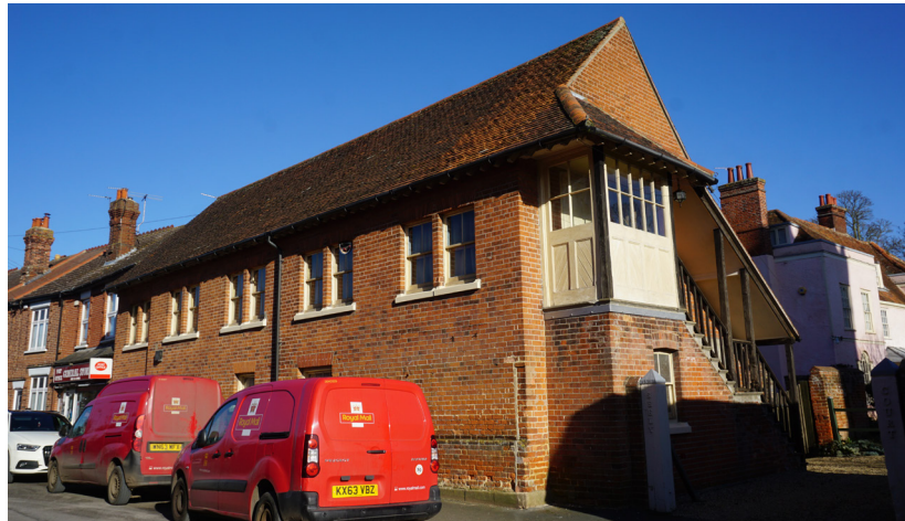
Figure 21 Church Hall (west of The Vicarage)
