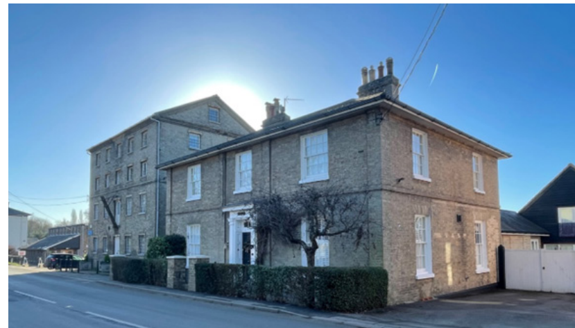
Figure 27 Mill House and Phoenix Mill
