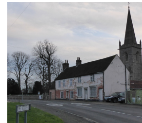
Figure 16 Grade II Listed 1 The Street (Church Cottage)
