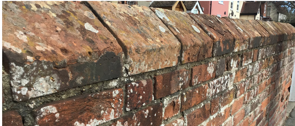
Figure 28 Brick wall with triangular section copings to the cottages along Thorpe Road
